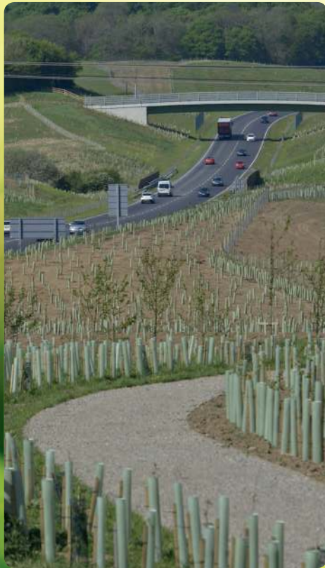
Accessed from the new Combe Valley Way
